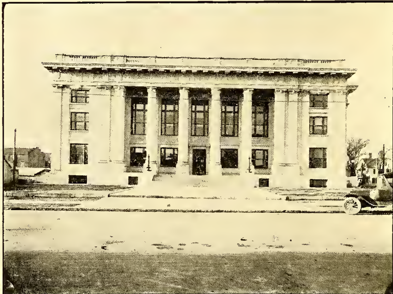
JOHNSTON COUNTY COURT HOUSE, SMITHFIELD, N. C.
